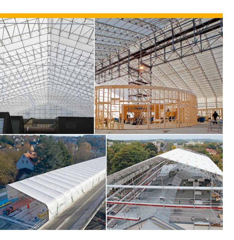
The Keder Roof XL is a lightweight, but very sturdy weather protection roof for great spans up to 40 m.
